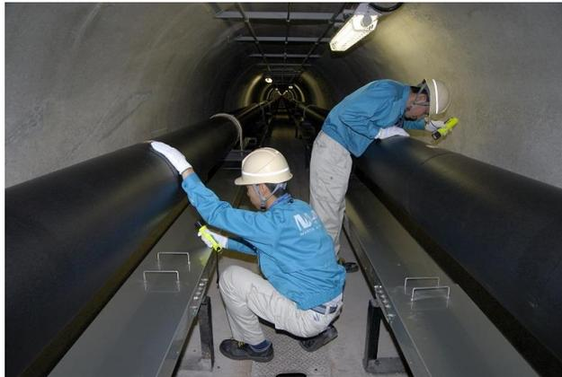
*Figure 33-Visual Inspection for Pipeline in the Tunnel Area*
