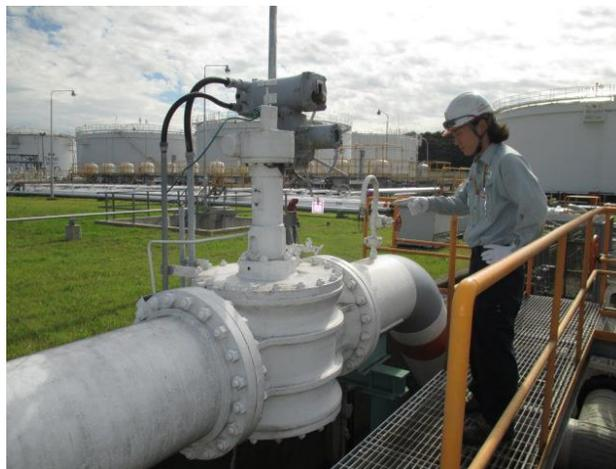
*Figure 35-Visual Inspection for Valves in the Storage Facility*
