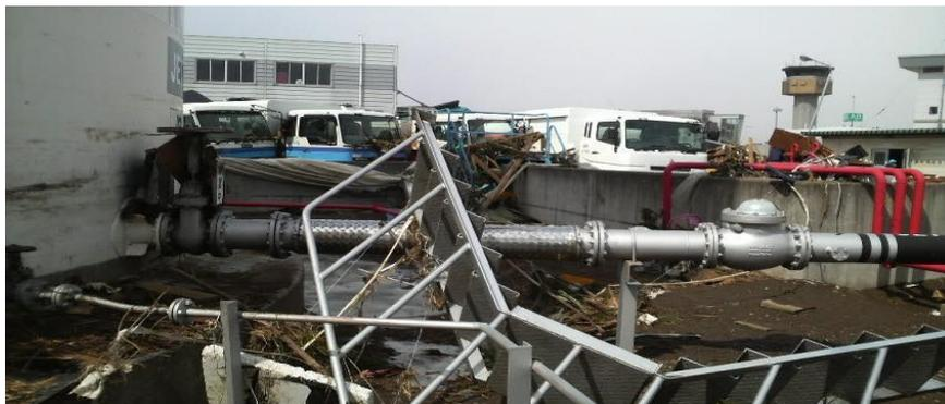
Figure 40-Photo showing less damaged tank and pipe and fell down steps
