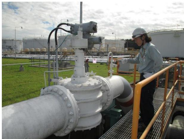
*Figure 35-Visual Inspection for Valves in the Storage Facility*
