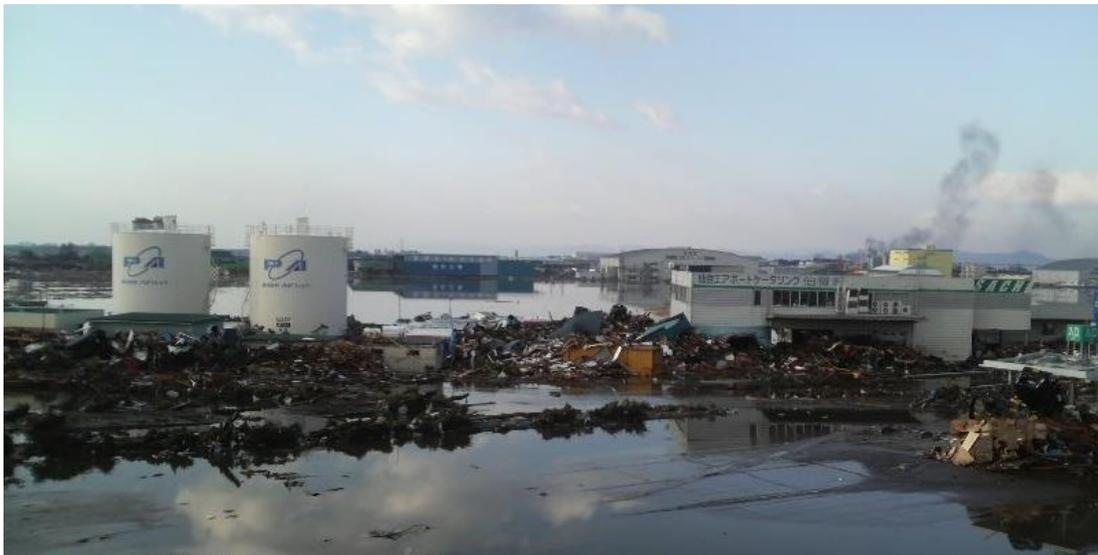
Figure 39-Photo showing huge volume of debris accumulated within fuel facility area
