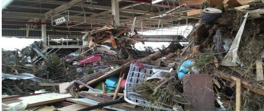
*Figure 41-Photo showing severely damaged and debris accumulated at fuel receiving bay and loading bay*
