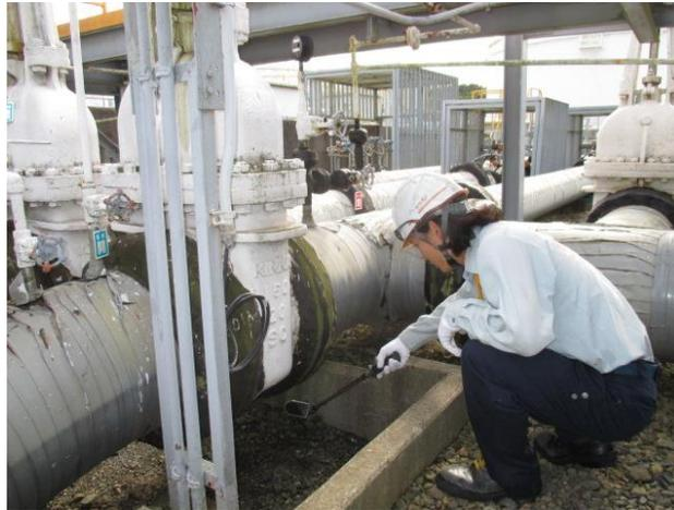
*Figure 34-Visual Inspection for Joint Area in the Storage Facility*
