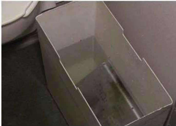
Figure 24 – The toilet waste bin with water holding the damaged device should be stowed and isolated in a toilet
